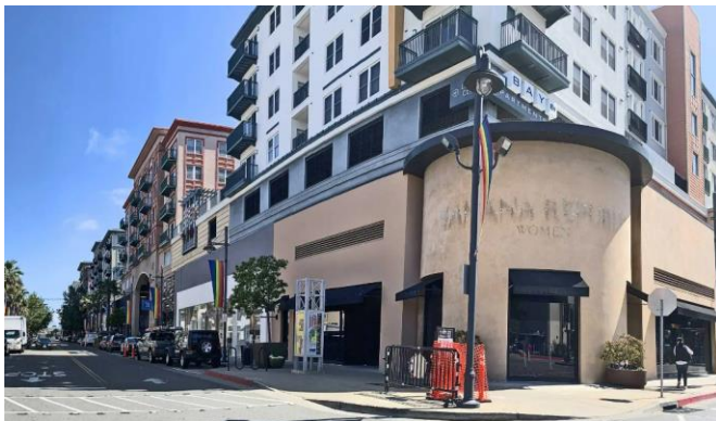
The former Banana Republic Women store at the Emeryville’s vacancy-filled Bay Street shopping center.
